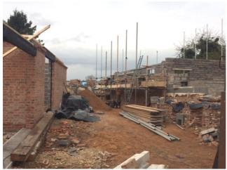
The Old School now has most of its ground floor lintels in place and the walls of the house are beginning to take shape.
