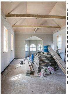
The builders, Trio are still cracking on at a pace and making a great job of it, the foyer, toilets and kitchen are all plastered and the kitchen units are being fitted as we go to press. The main hall has to be plastered with lime plaster - a three layer process. It has to cure between layers. The first coat had been applied when these photos were taken. Trio's expectation to finish is still by the end of July and we can't wait to see it.
