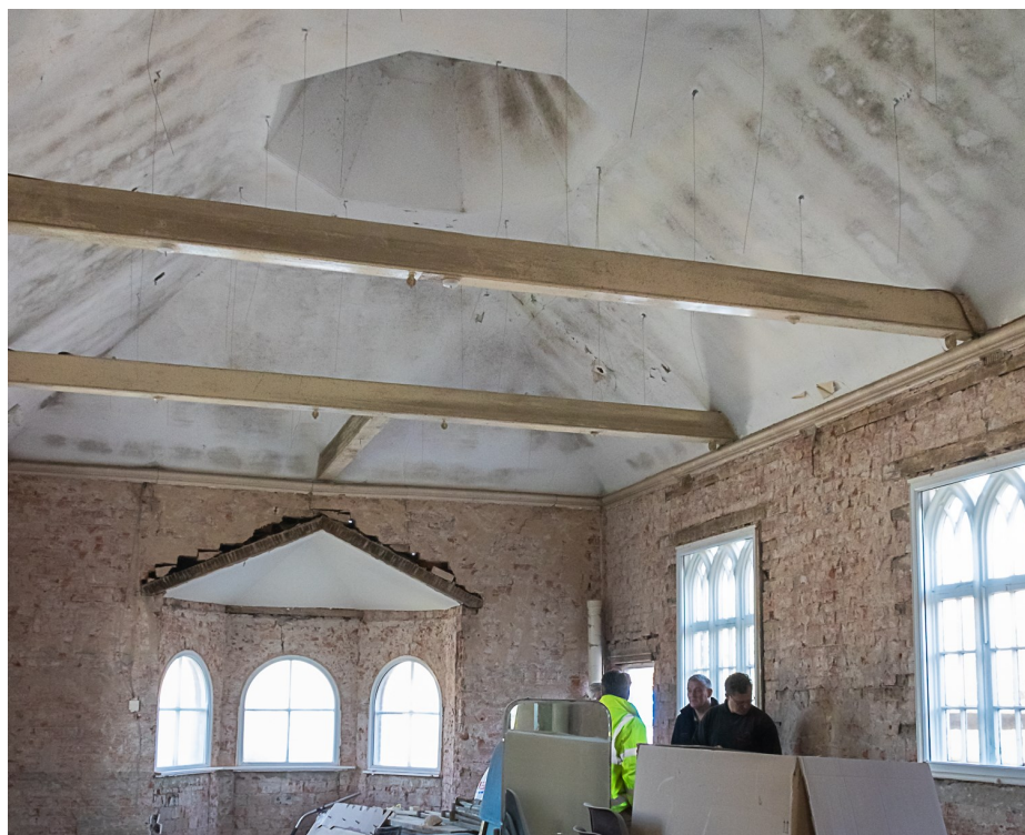
The Laxton Village Hall Stripped of False Ceiling and Plaster, 26th February 2019
